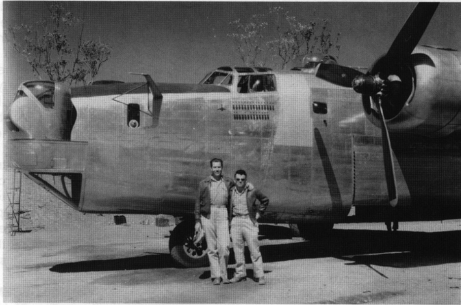
Another "J" model B-24, but this one has braced pitot tubes on both sides, no side windows to the bombardier compartment and the earlier, A6A hydraulic nose turret. A. V. Connery Collection
