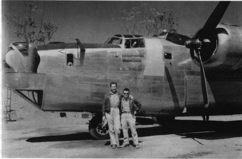
Another "J" model B-24, but this one has braced pitot tubes on both sides, no side windows to the bombardier compartment and the earlier, A6A hydraulic nose turret.
