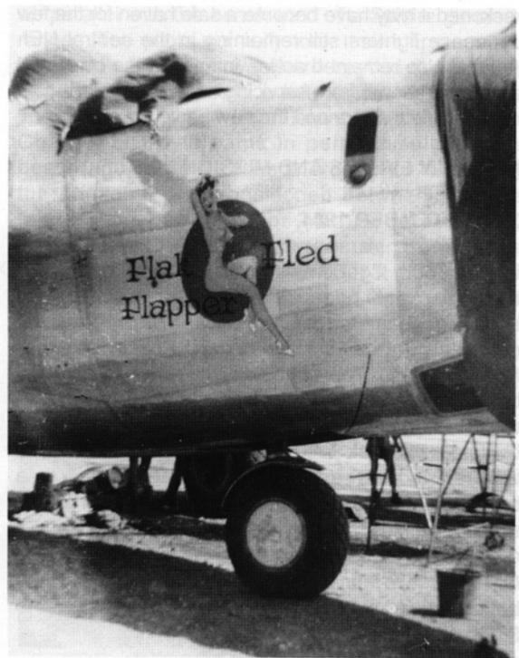
Note the lack of external nose wheel doors indicating the ship has a hydraulically powered nose turret.
