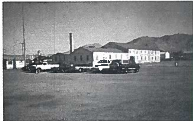
Operations Area Buildings
