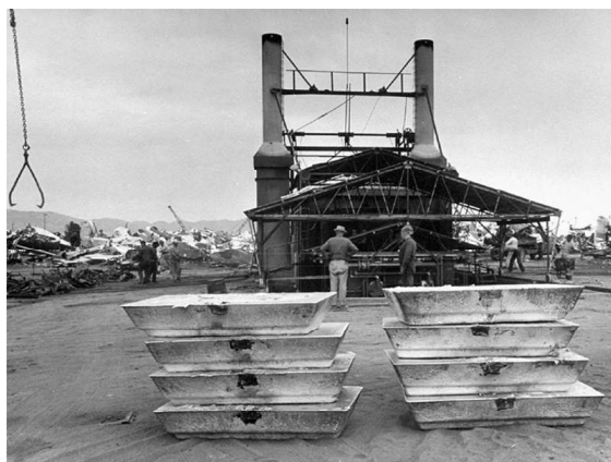
Kingman, AZ, boneyard Smelter. This is where the scrapped aircraft went to be melted down.
