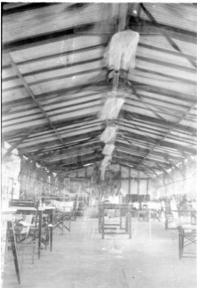
Interior of our Red Cross Building
