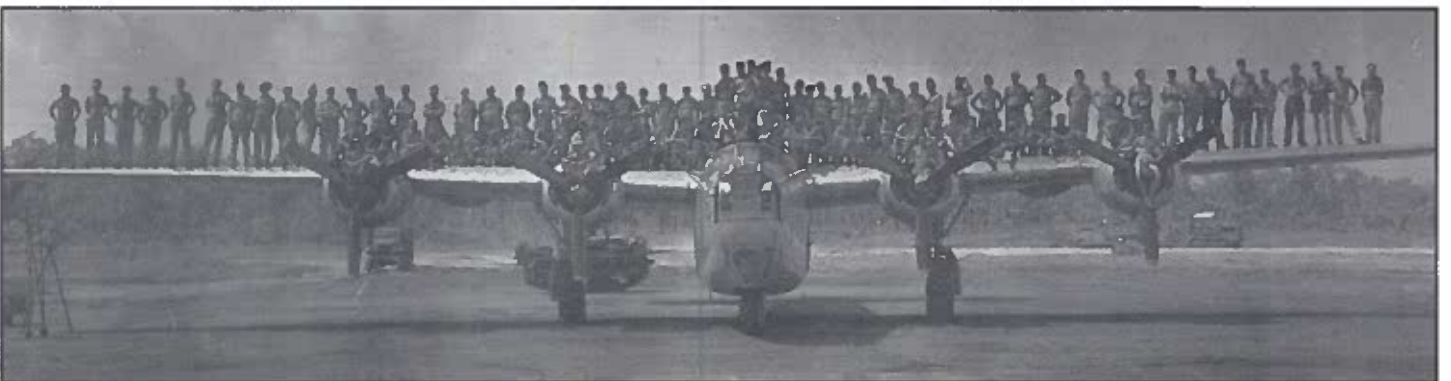
529th Engineering and Maintenance Staff
